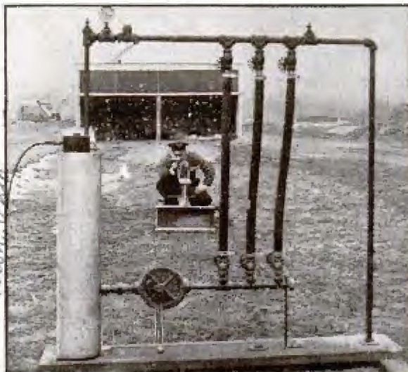
Above, testing samples of synthetic and natural rubber for their resistance to sunlight with a machine that produces ultraviolet light in laboratories of the U. S. Rubber Co. Synthetics show a high rate of resistance
